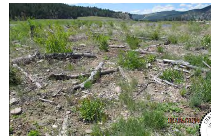
EXAMPLE OF CONSTRUCTED FLOODPLAIN ROUGHNESS
